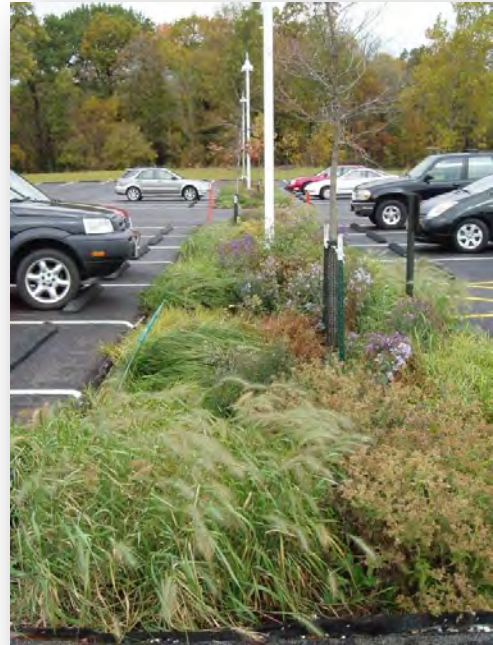
Bioswales in parking lots help filter stormwater runoff. This one is at the Ryerson Woods welcome center – USGBC-certified LEED Platinum.
